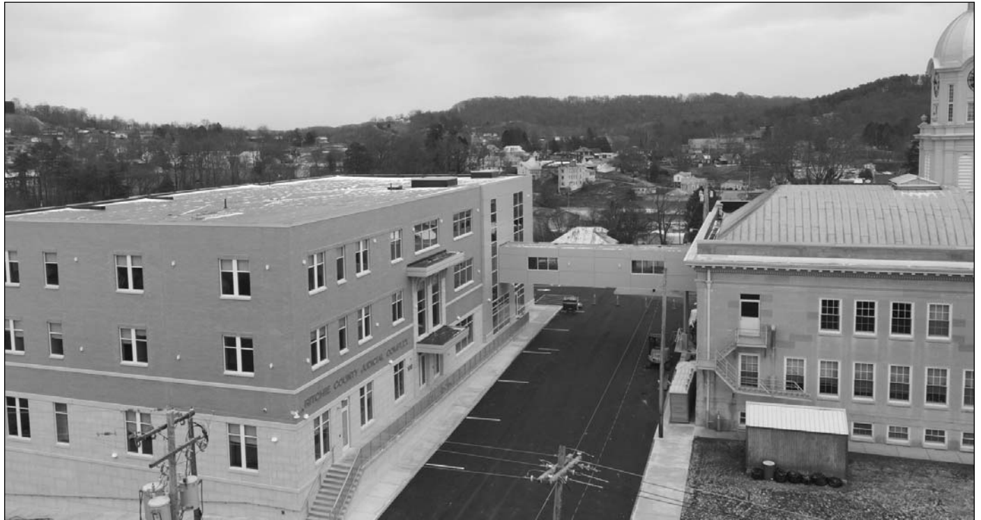
An aerial view of the newly completed Ritchie County Judicial Complex building with a walkway to the older Ritchie County Courthouse. A ribbon cutting and open house was held for the new building earlier this month.
