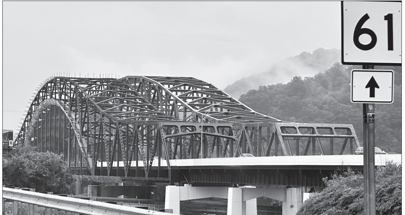
The Chuck Yeager Bridge in Kanawha County, WV was the site of two separate incidents, involving more than ten vehicles, which were struck and damaged by unsecured cables on a nonunion bridge painting project last month.
