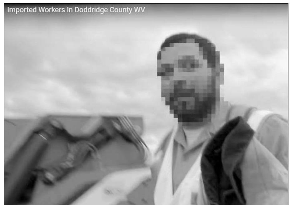
Construction workers from Guatemala and Mexico were working at the Clearwater facility in May of 2017. The $300 million water treatment plant in Doddridge County was temporarily shut down in September.
