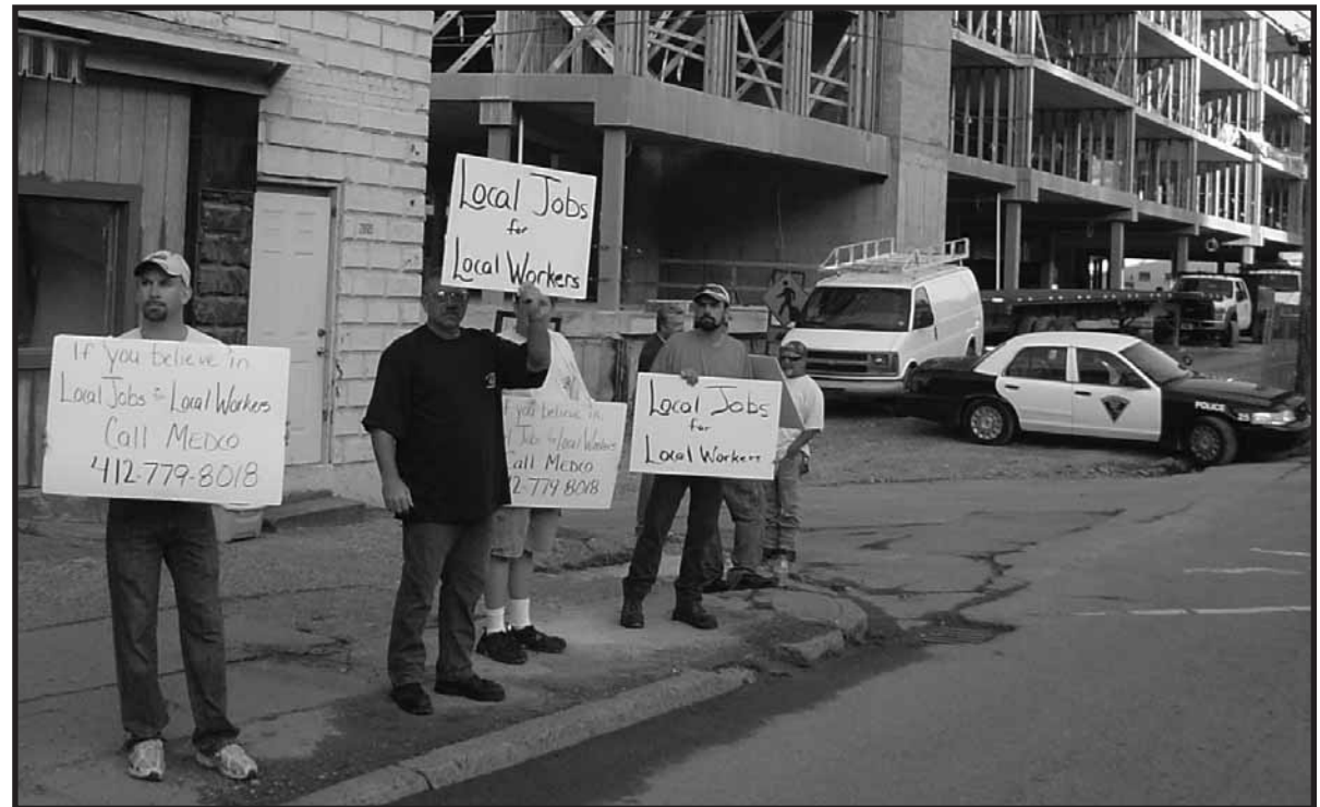
MEMBERS OF THE Carpenters let the public know the Beech View Place project in Morgantown, made possible with local Tax Increment Financing, ended up creating jobs for out-of-state companies and workers.
