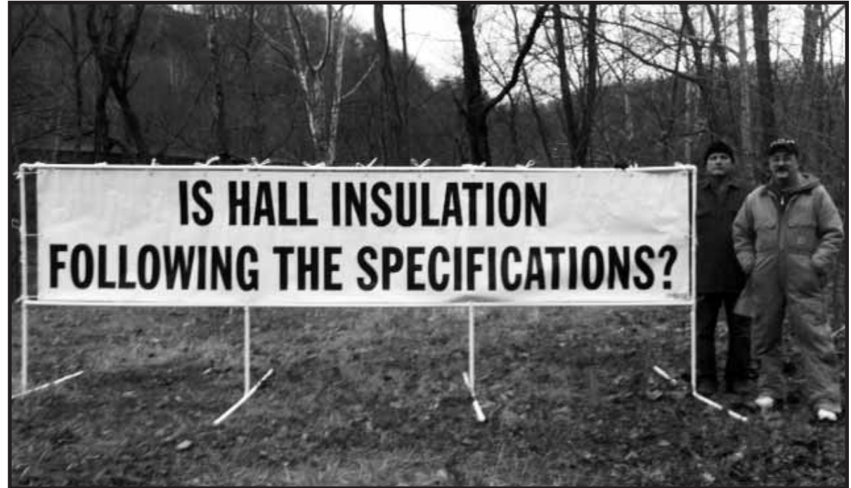
USING A BANNER to raise awareness about possible specifications issues are Insulator Agent Mike Loeffert, and insulator mechanic Ric Jones of Kingwood, WV at the Camp Dawson site in Preston County.
