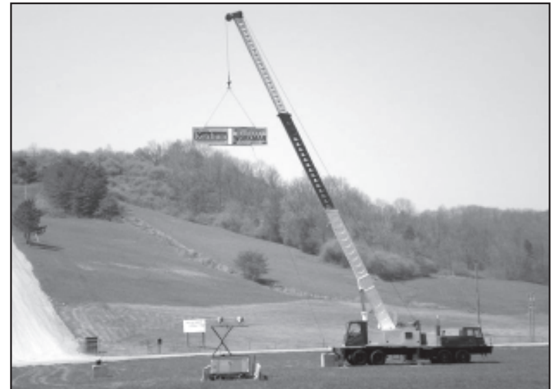
OPERATING ENGINEERS 132 used a crane to raise two large signs supporting WV Supreme Court endorsed candidates Menis Ketchum and Margaret Workman.
