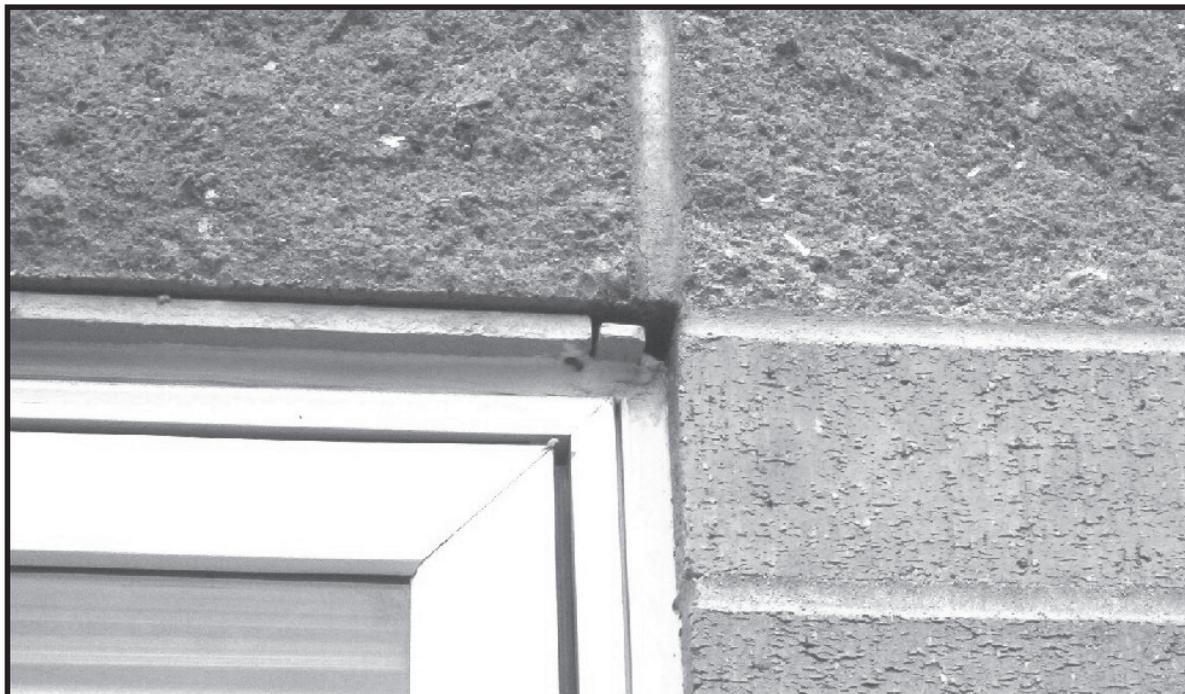
**THIS PICTURE SHOWS a lintels that is too short. It was installed by Lang Masonry and is just one of many examples of shoddy work found and documented at the Frontier High School.**
