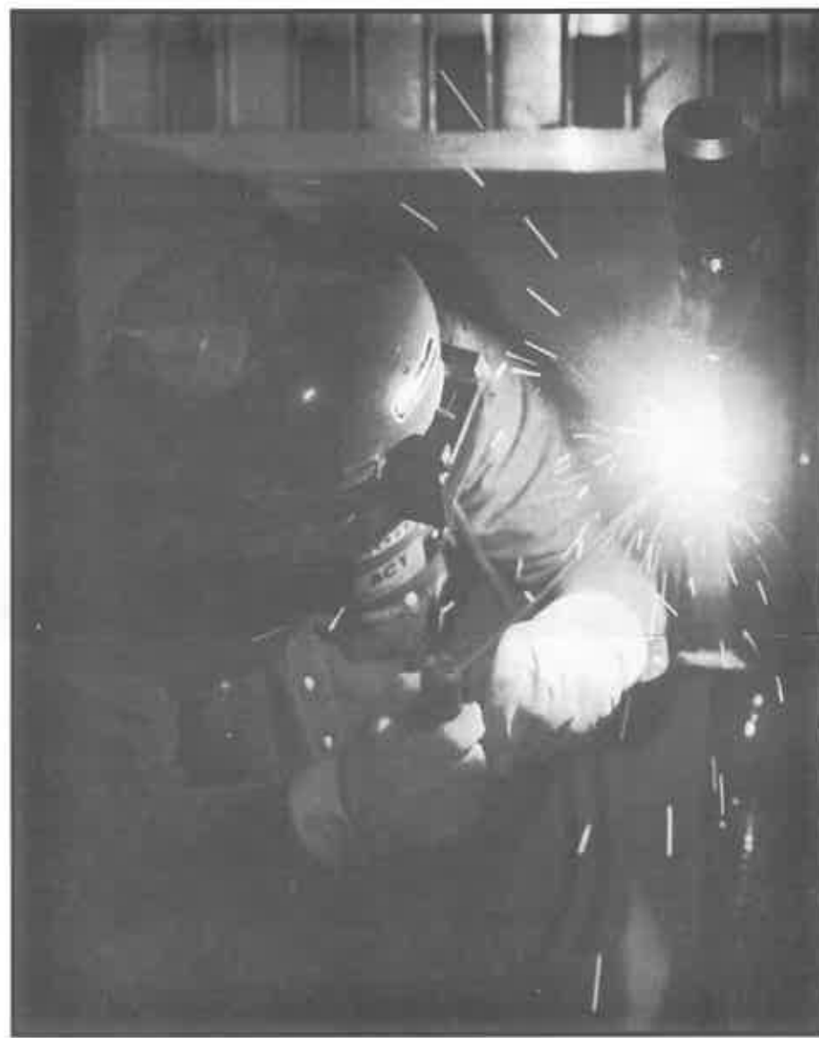
KURT HAMRICK OF BOILERMAKERS LOCAL 667 is pictured checking the heat on his machine as he prepares for testing as part of the Common Arc program.
