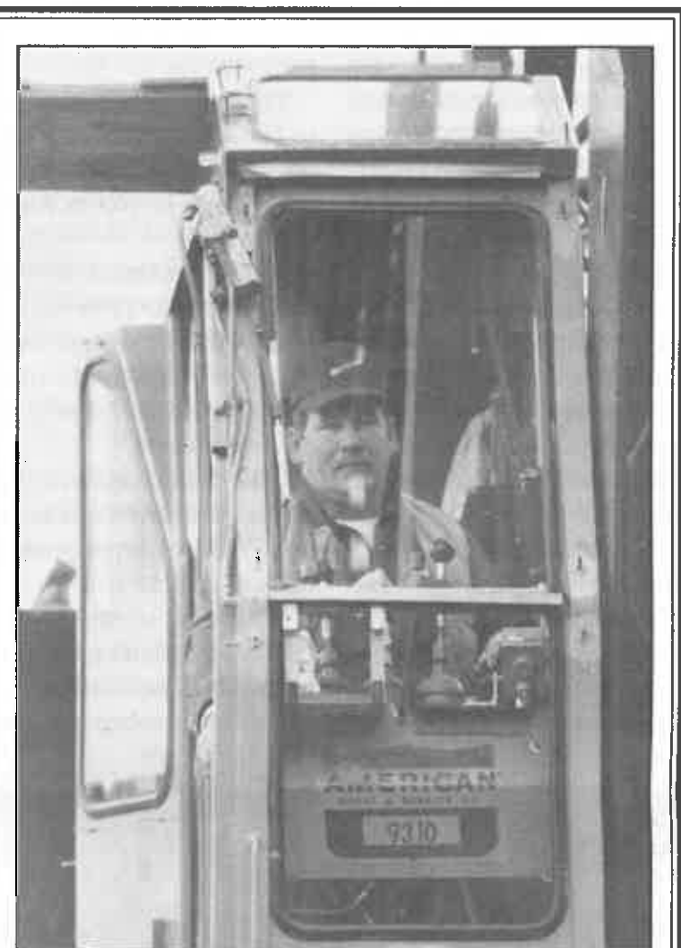
IN THE BUCKET on Gorridor G near Logan is Gary McClanahan of St. Albans. McClanahan and four other members of Operating Engineers 132 are working on the project building a bridge over the Mud River.
